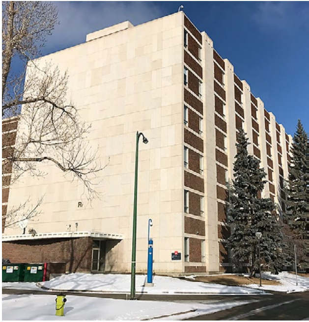
Figure 14. SAIT; This is the south side of the Senator Patrick Burns Building, entirely clad with white, fossiliferous Tyndall Stone.
