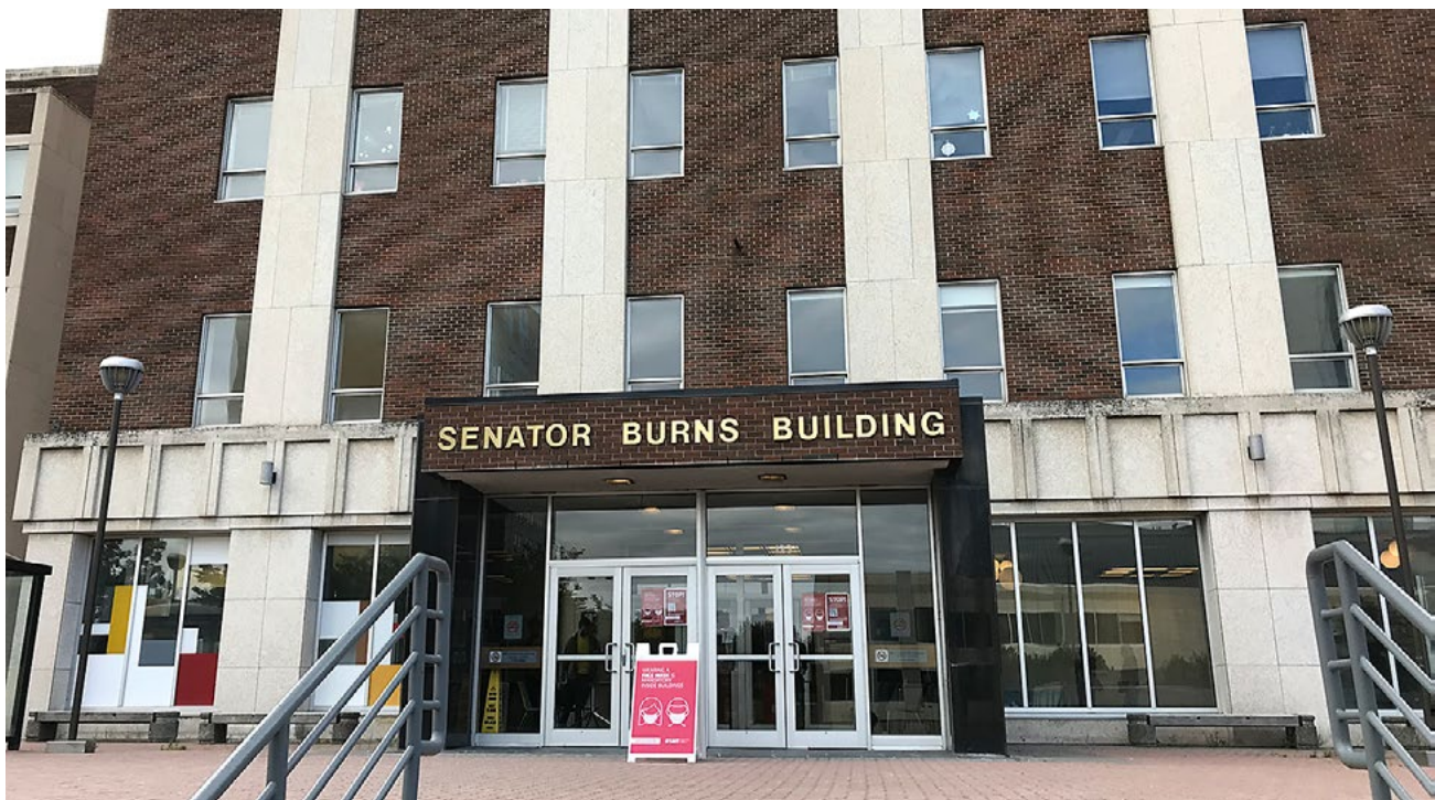
Figure 13. SAIT; north entrance to the Senator Patrick Burns Building which was built in 1967. The white columns are Tyndall Stone. The slabs have been subject to 53 years of weathering but show very little signs of deterioration, allowing the numerous fossils to be clearly viewed.
