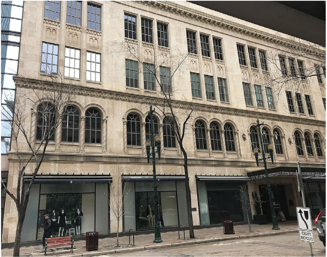
Figure 3. South-facing front of the former Eaton's building (currently Hy's Steakhouse), on 8 Avenue between 3 Street and 4 Street SW, entirely clad in Tyndall Stone.
