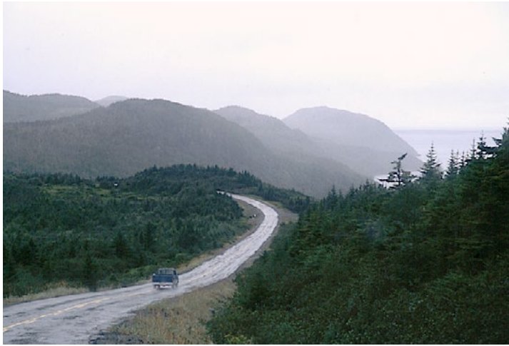
Figure 29. Wet and foggy highway near Fox Harbour.
