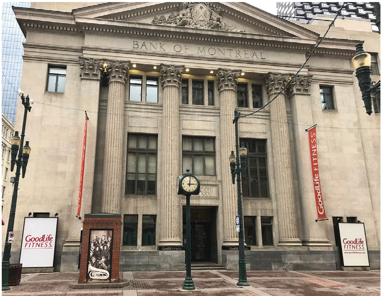
Figure 1. The entrance to the Bank of Montreal Building (currently Goodlife Fitness) on the northeast corner of 1 Street and 8 Avenue SW, (Stephen Avenue Mall), the columns and façade are entirely Tyndall Stone.
