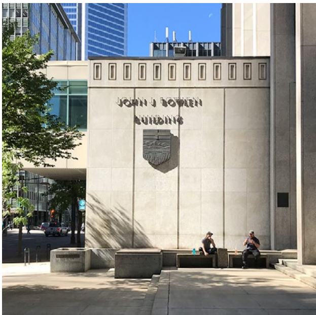
Figure 4. Entrance to the John J. Bowlen Building, former Calgary Court House Building, 620 7 Ave. SW. Built in 1969, inaugurated by Premier Harry J. Strom. White blocks are Tyndall Stone.
