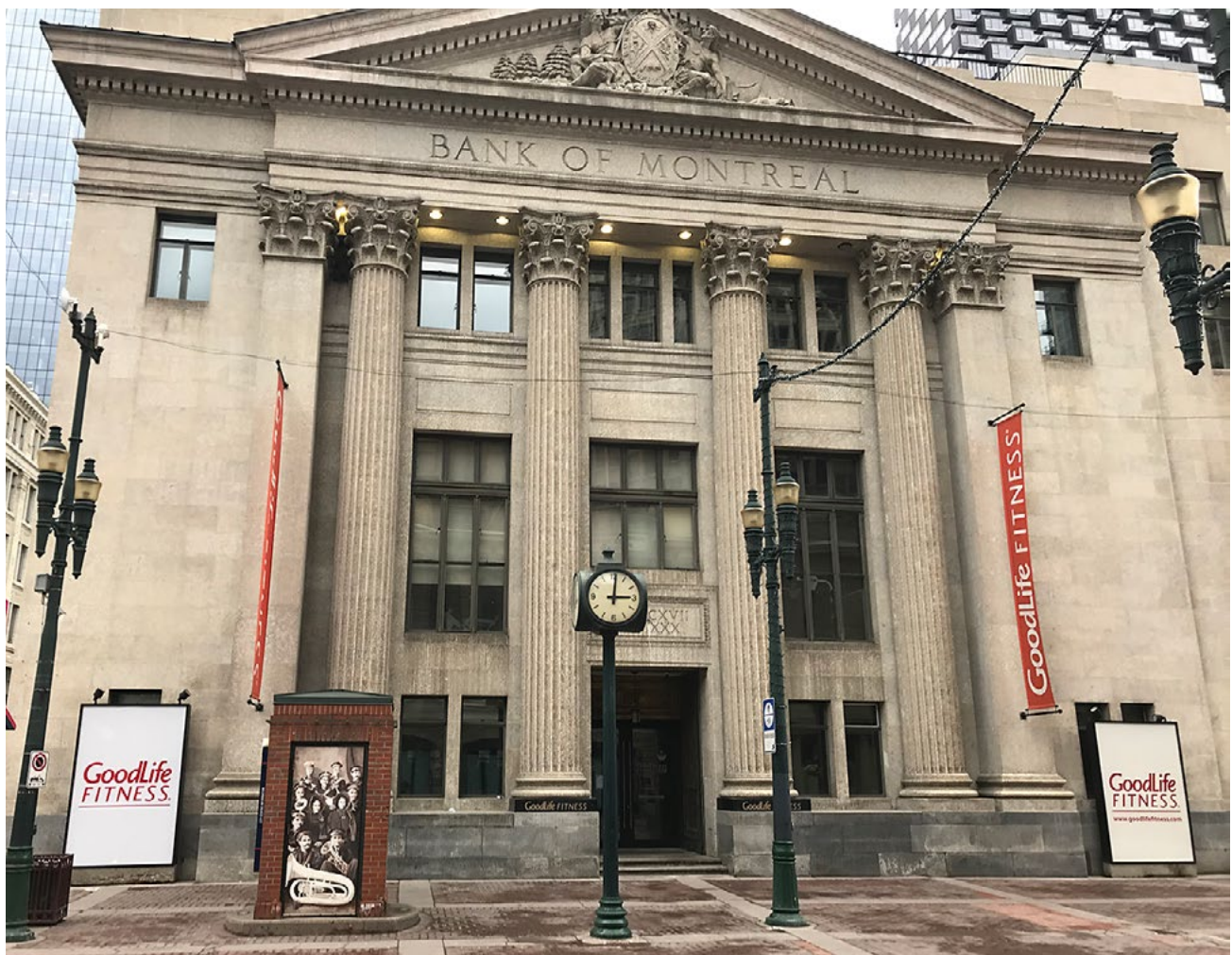
Figure 1. Front of the Bank of Montreal Building (now Goodlife Fitness) on the northeast corner of 1st Street and 8th Avenue S.W. (Stephen Avenue Mall), in downtown Calgary. The columns and façade are entirely Tyndall Stone. Photo by Tako Koning.
