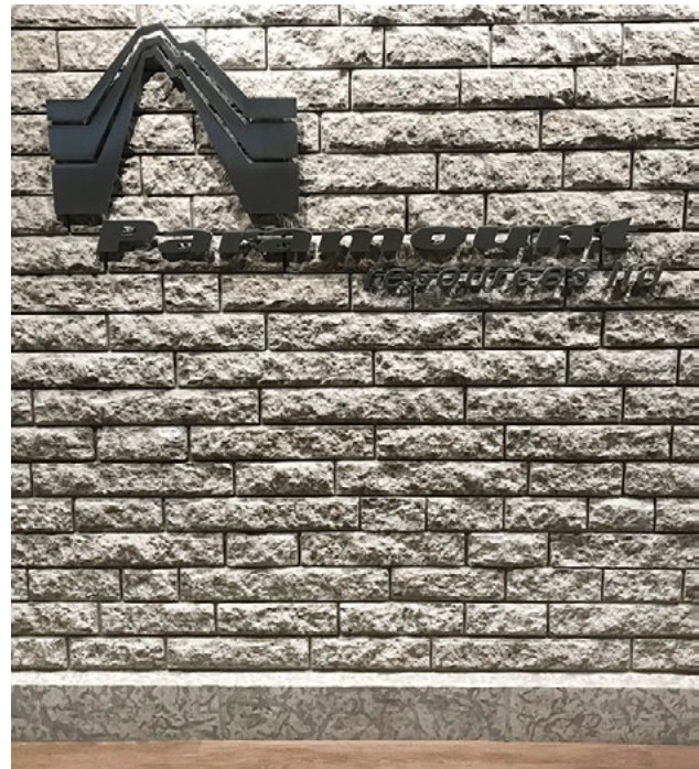
Figure 1. Rough cut Tyndall Stone clads the entrance to Paramount Resources corporate office on the 47th floor of Bankers Hall.
